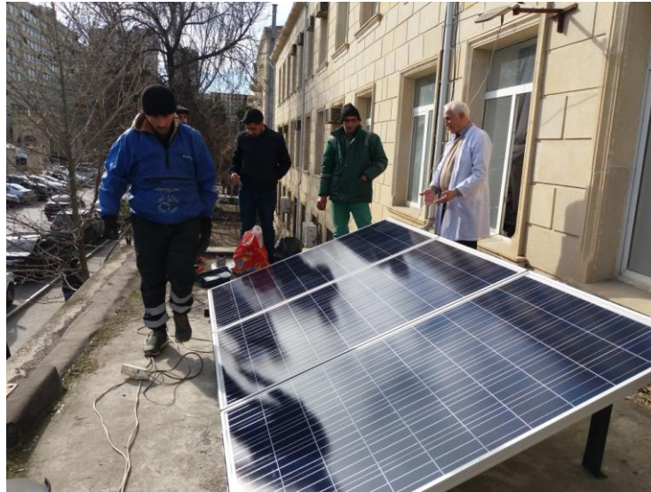
Figure 1. General view of the SPCS, with a power of 750 W, mounted on the facade at the entrance of the Institute of Radiation Problems under the MSE of the Republic of Azerbaijan
